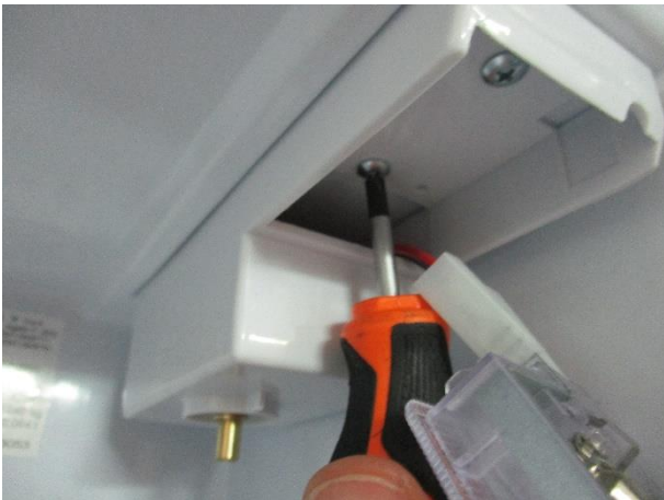
9. Unscrew the protection box (2 bolts)
